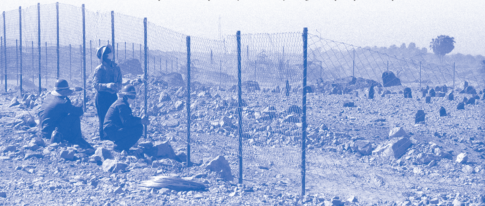
SUDAN: Chinese workers at the Merowe Dam site. Photo: David Haberlah
